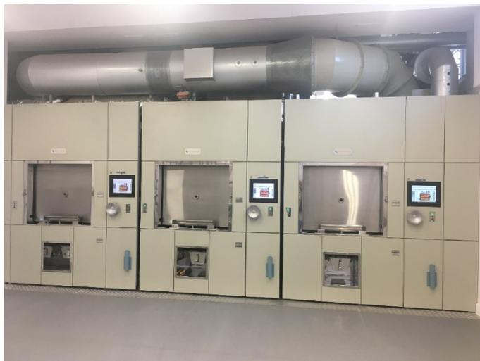
The decision was taken to line the new cremators with refractory bricks which are more durable than conventional linings, they retain more heat in the brickwork resulting in less gas usage, and the cremators are fitted with smart software that monitors the conditions in the cremators and maintains the required temperature to meet operating conditions.
