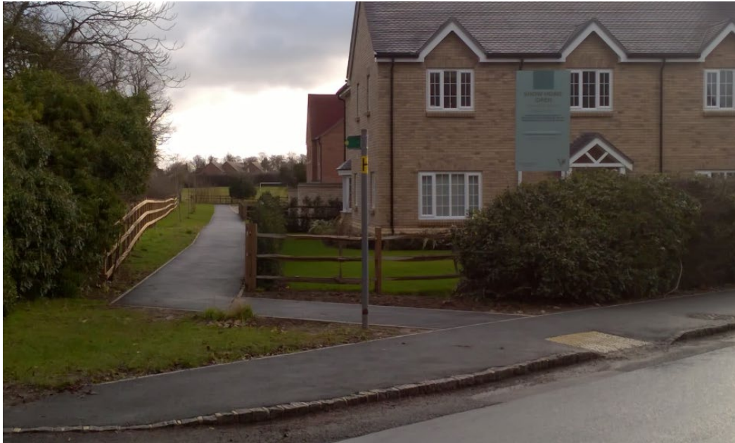
Fig. 3 - bitumen-surfaced footpath and dropped kerb serving new residents with a route to school and access to green space in Stone
