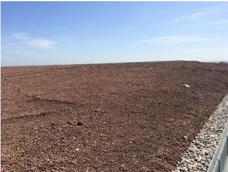
April 2016, during installation of the first green roof.
