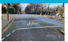
A stop line for cyclists at traffic signals marked beyond the stop line for general traffic. This helps bring priority to cyclists as they pull away in front of traffic. It also helps avoid conflict with vehicles turning.
