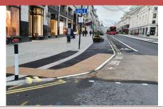
A section of footway extended out into the carriageway to reduce the crossing distance and improve visibility.
