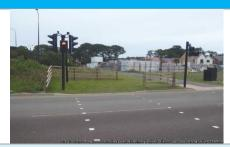
A signal-controlled crossing for horse-riders, pedestrians and cyclists using signal heads and a flashing light crossing period that is push demanded at a level for horse riders.
