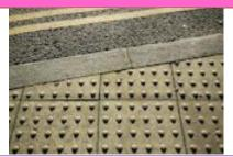
Dropped kerbs facilitate non stepped access, usually between the footway and carriageway. These should be accompanied by tactile paving, which provides a distinctive, raised surface profile to be detected by both sighted and visually impaired users.
